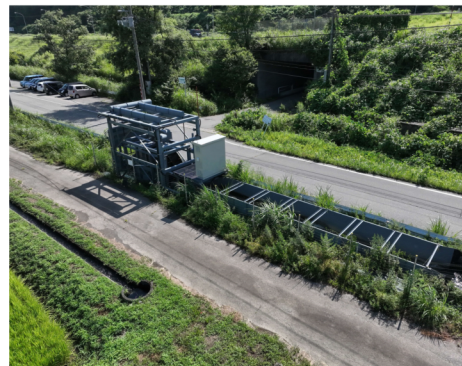
On site test1
